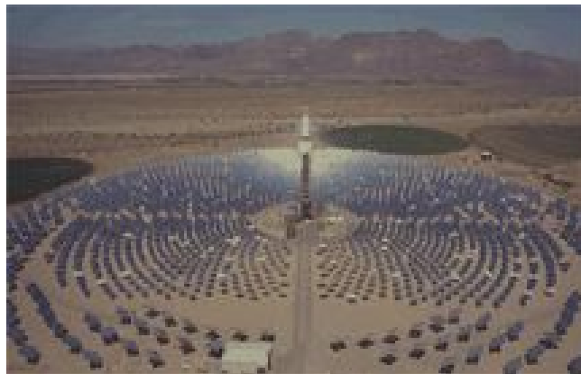
Hundreds of curved reflectors focus the sun’s energy to a central tower.
